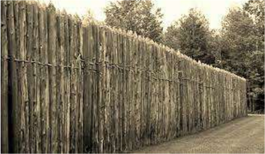
Figure 3. Example of a palisade constructed as a defensive structure. (Photo Credit: http://www.uk-archaeology.tv/ )
